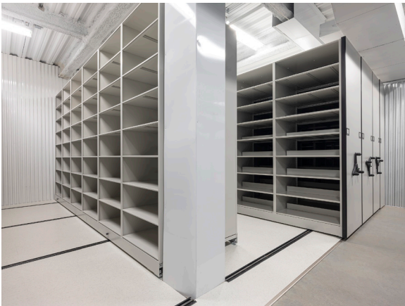
A private room at UOVO: NYC feature high-density racking
